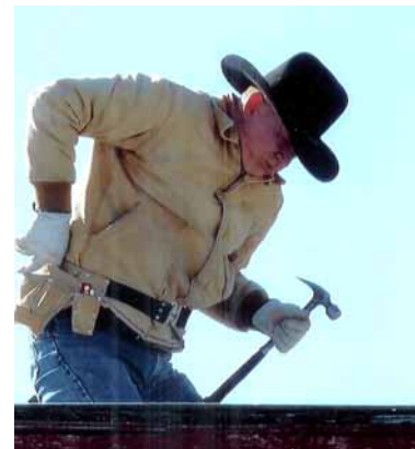
Terry Michel (Mr. Fixit) built a much needed shed and repaired other wind damaged sheds
